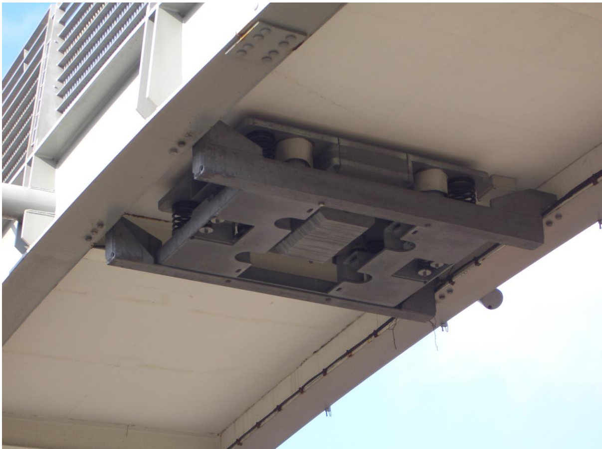
Photo 2 – Tuned Mass Damper Installed Under Bridge Deck
