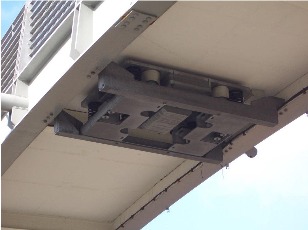
Photo 2 – Tuned Mass Damper Installed Under Footbridge Deck
